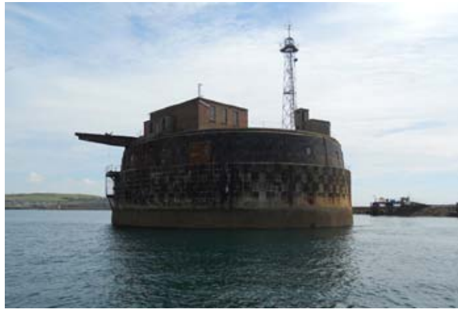
Breakwater Fort Plymouth Sound. The Crown Jewels lies a few metres from the fort wall in the centre of the picture. Nikon Coolpix S3000, auto.
